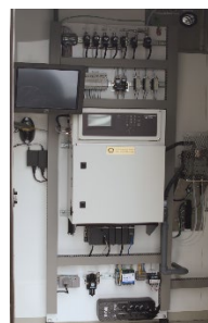
Standalone system cabinet or Panel with MC3 analyzer, PLC and sample system components
